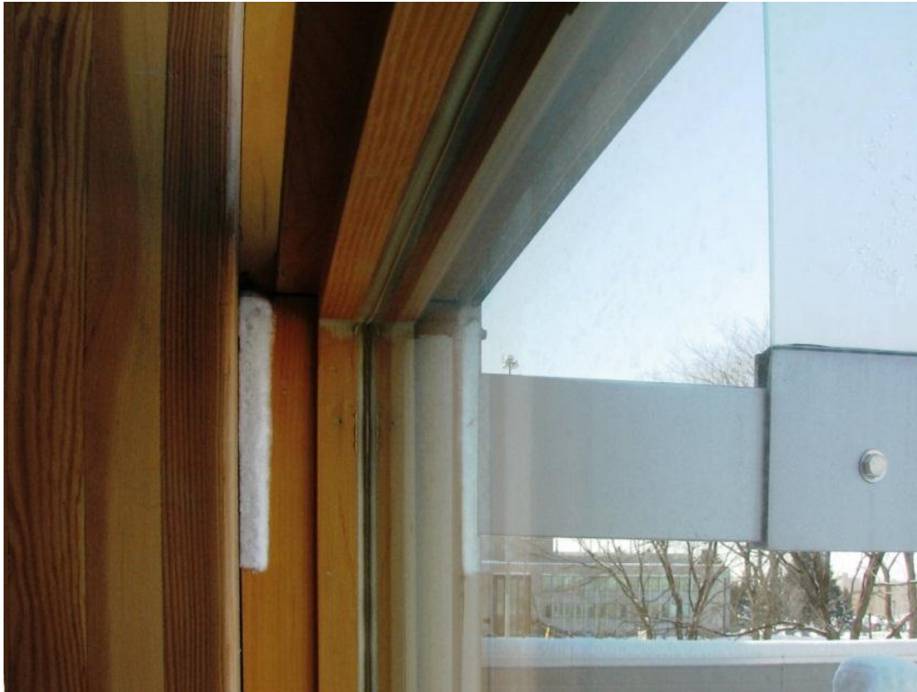
Figure 20: Thermal bridge before putting insulating material on the metal component of the sun shading device
